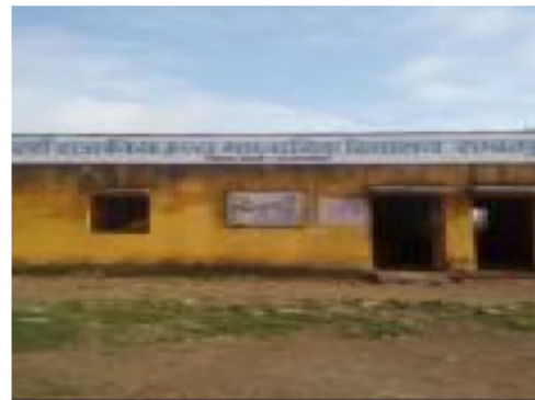
Building Front View
