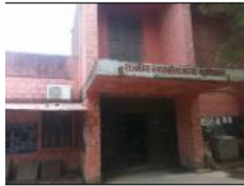
Building Front View
