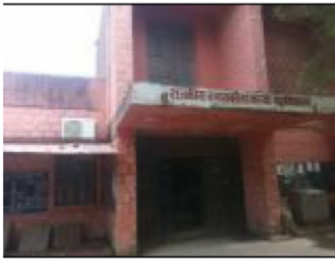
Building Front View
