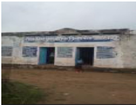
Building Front View
