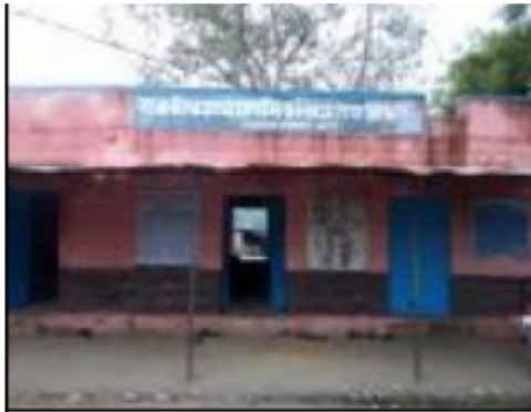
Building Front View
