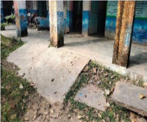
Polling Station Building Front View
