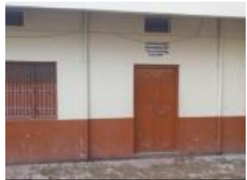
Building Front View
