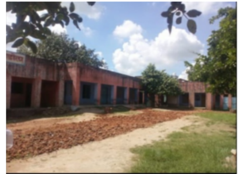
Building Front View
