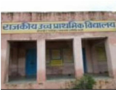
Building Front View
