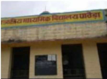
Building Front View
