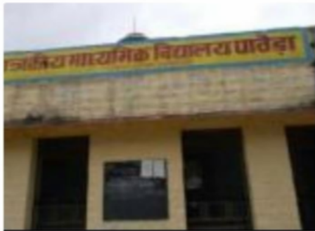
Building Front View
