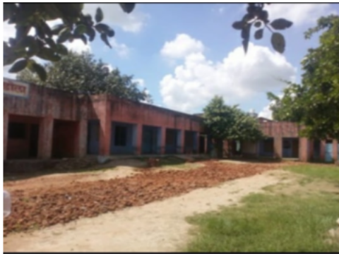
Building Front View
