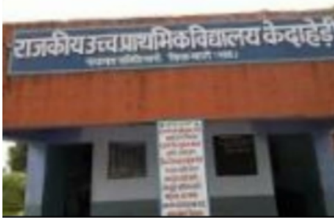
Building Front View
