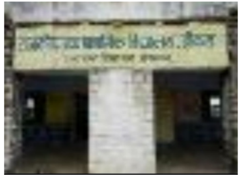
Building Front View
