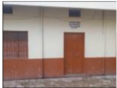
Building Front View
