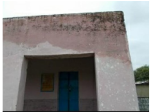
Building Front View
