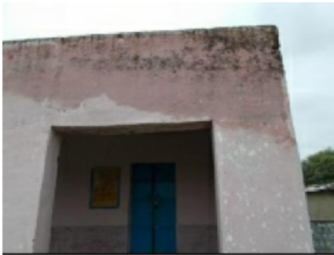
Building Front View
