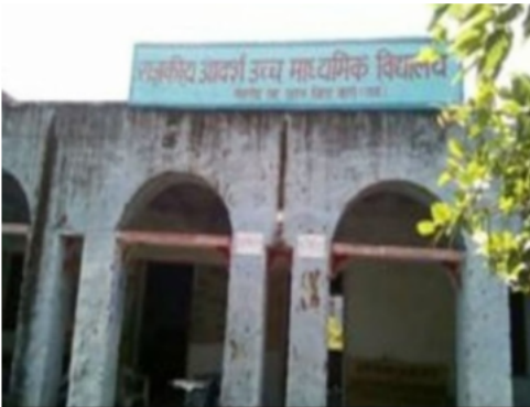
Building Front View
