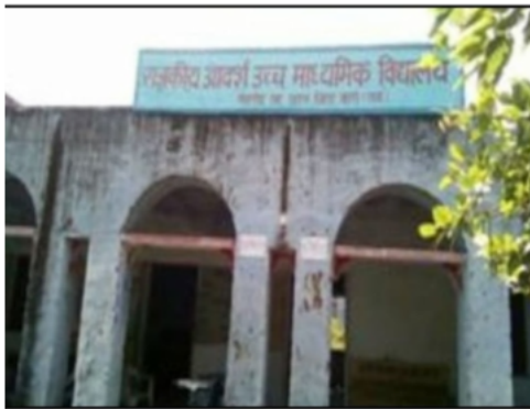
Building Front View
