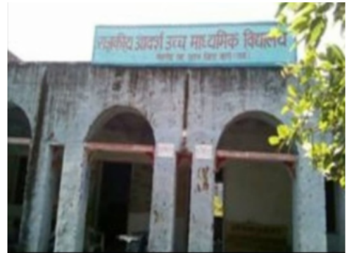
Building Front View
