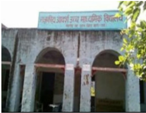
Building Front View
