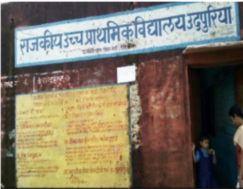
Building Front View
