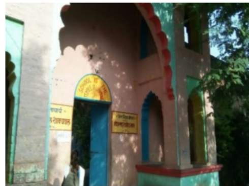
Building Front View
