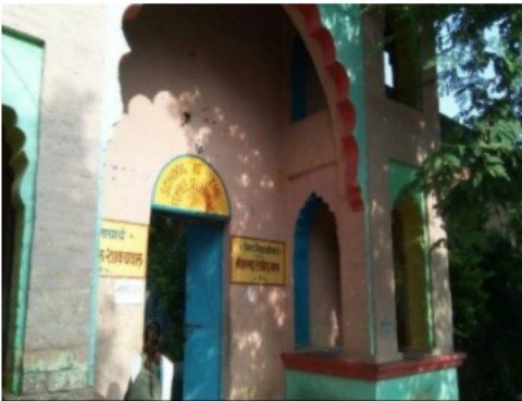
Building Front View
