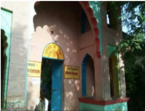
Building Front View
