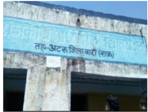
Building Front View
