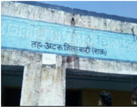
Building Front View
