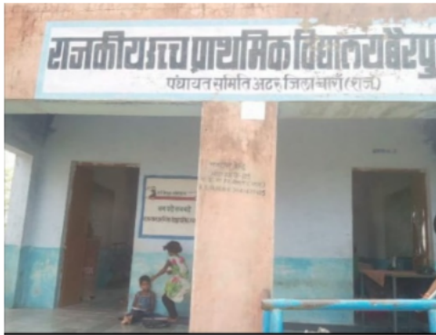
Building Front View
