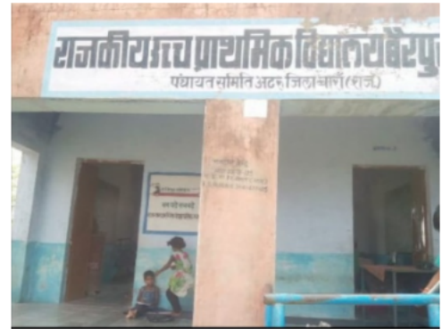
Building Front View
