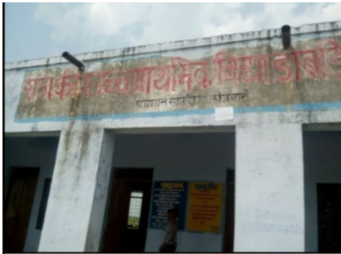
Building Front View
