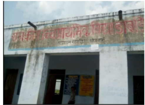
Building Front View
