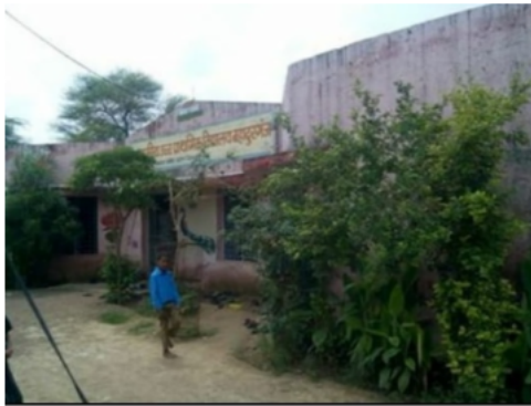
Building Front View
