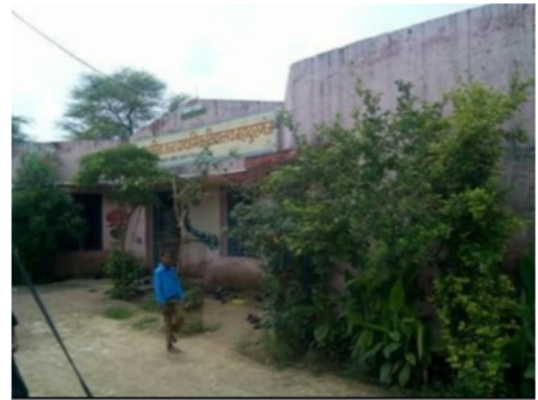
Building Front View
