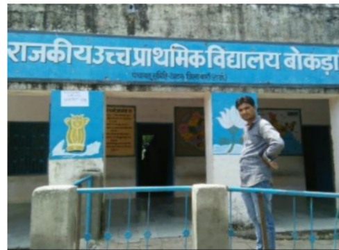
Building Front View
