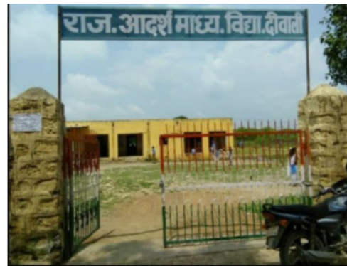
Building Front View
