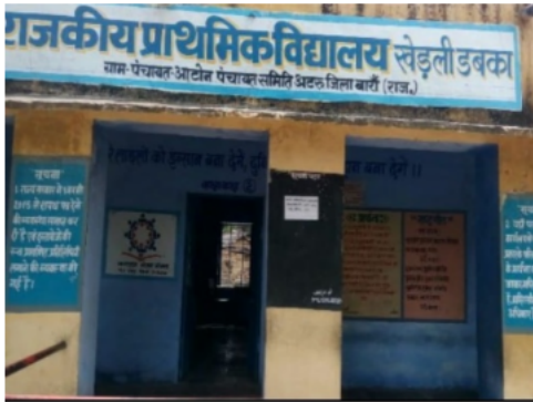
Building Front View
