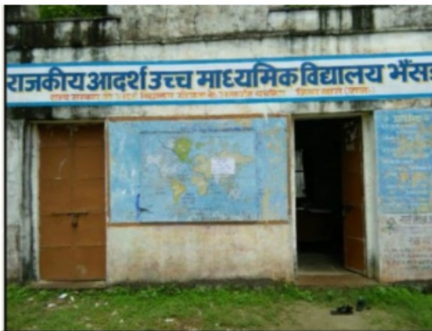
Building Front View
