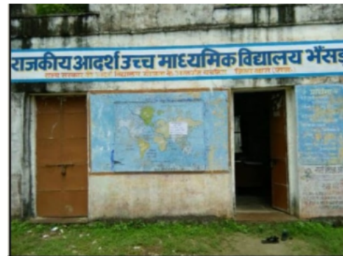
Building Front View
