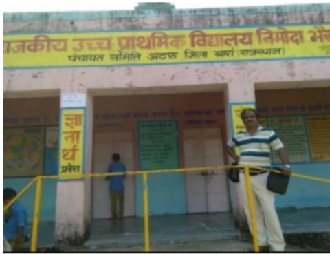
Building Front View
