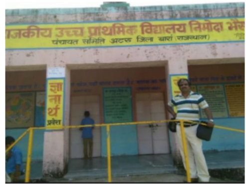
Building Front View
