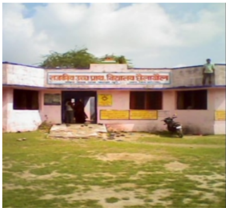
Building Front View
