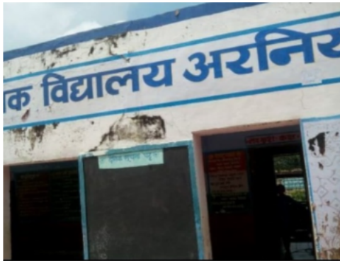
Building Front View
