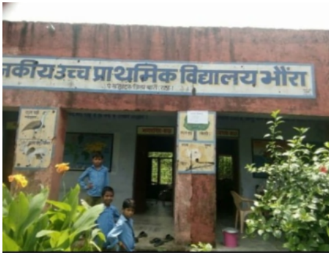
Building Front View
