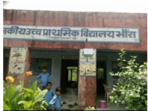
Building Front View
