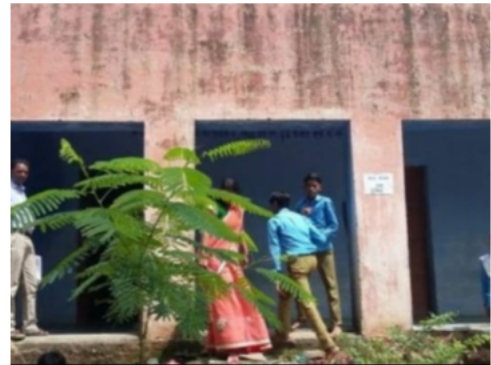
Building Front View
