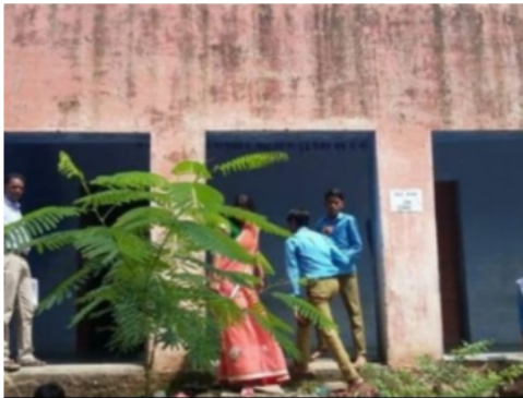
Building Front View
