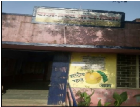
Building Front View
