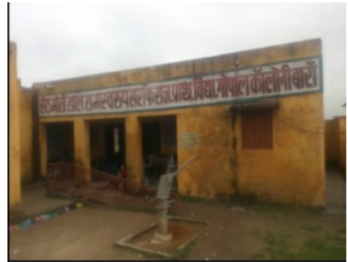
Building Front View
