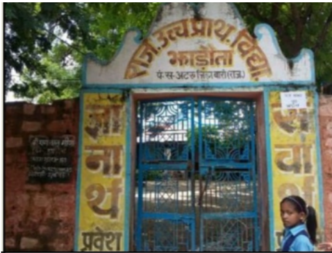
Building Front View
