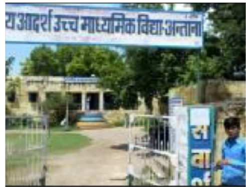
Building Front View
