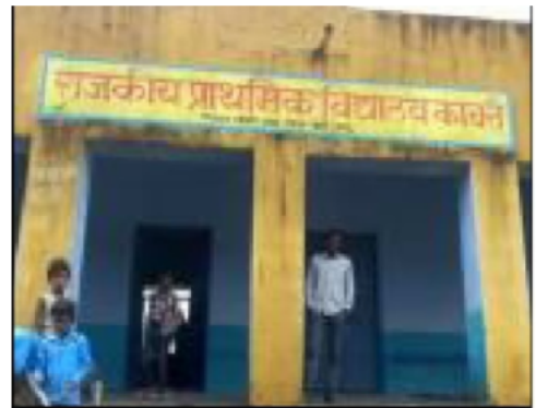
Building Front View
