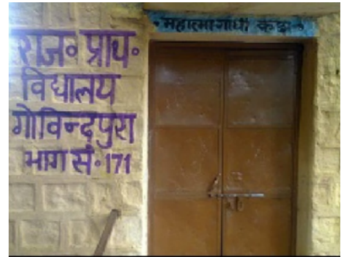
Building Front View
