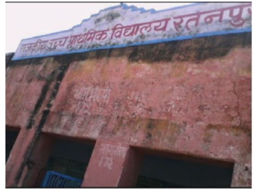
Building Front View
