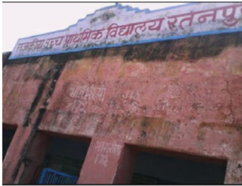
Building Front View
