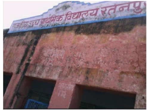
Building Front View
