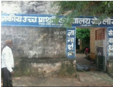
Building Front View
