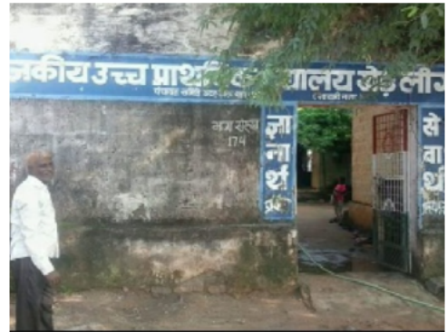
Building Front View
