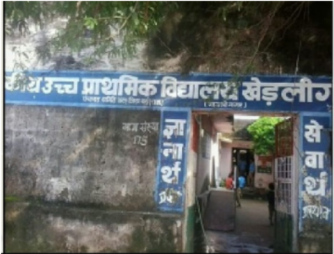
Building Front View
