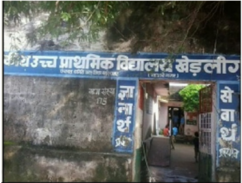
Building Front View
