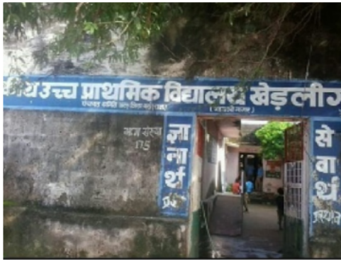
Building Front View
