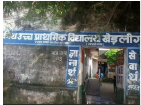
Building Front View
