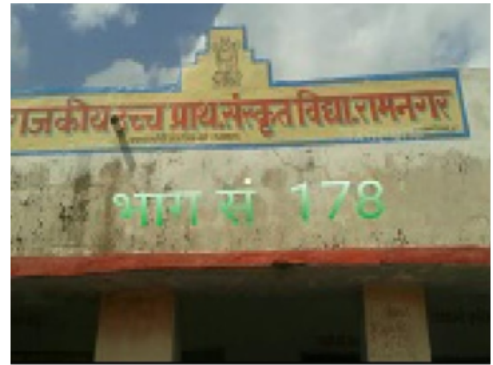
Building Front View
