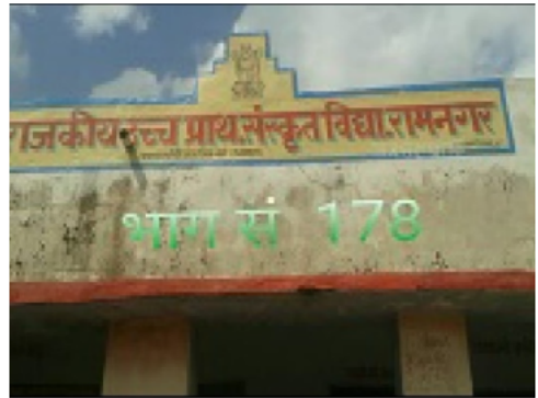
Building Front View
