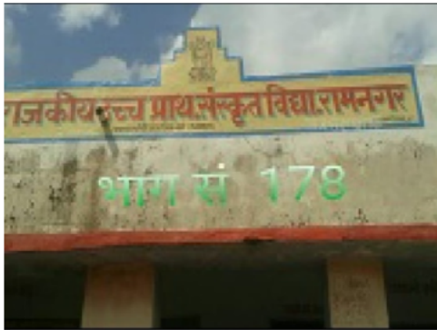
Building Front View
