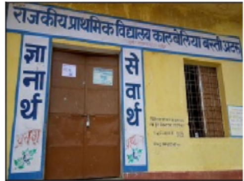
Building Front View
