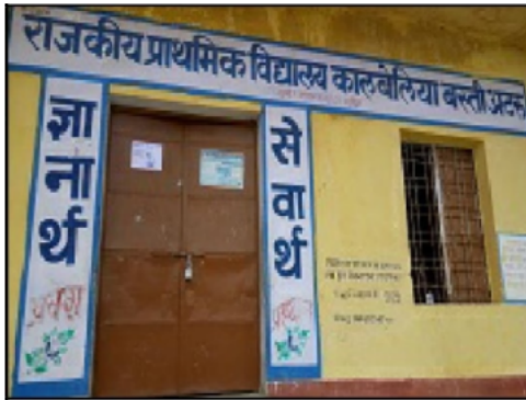
Building Front View
