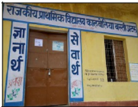
Building Front View
