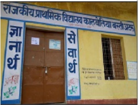
Building Front View
