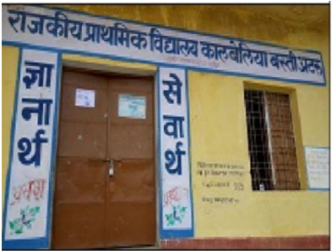
Building Front View
